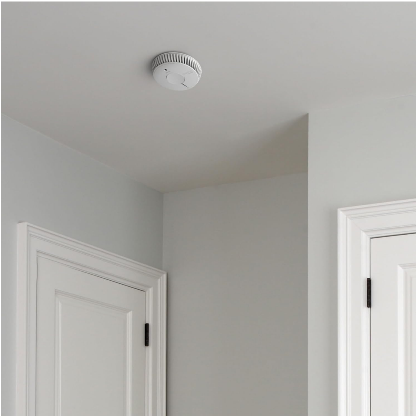
Image: An AngelEye smoke detector mounted on a white ceiling in a residential hallway, demonstrating a typical installation location.
