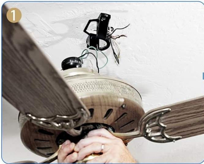
1 Disconnect the ceiling fan wiring
