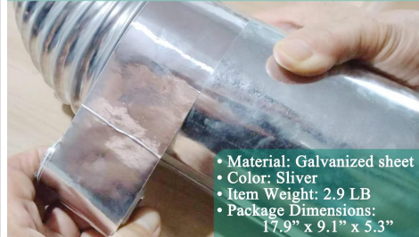
Image: Demonstrates the proper application of aluminum foil tape for sealing vent connections.
