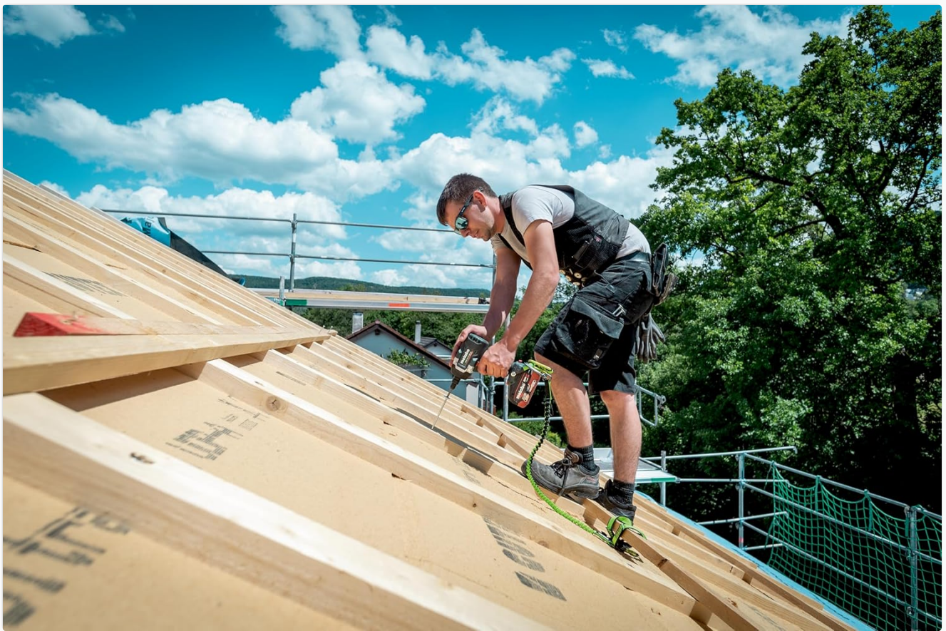
Figure 4: A worker utilizing the Metabo impact wrench for fastening on a roof structure. This demonstrates the tool's application in construction environments, highlighting its portability and power for overhead work.
