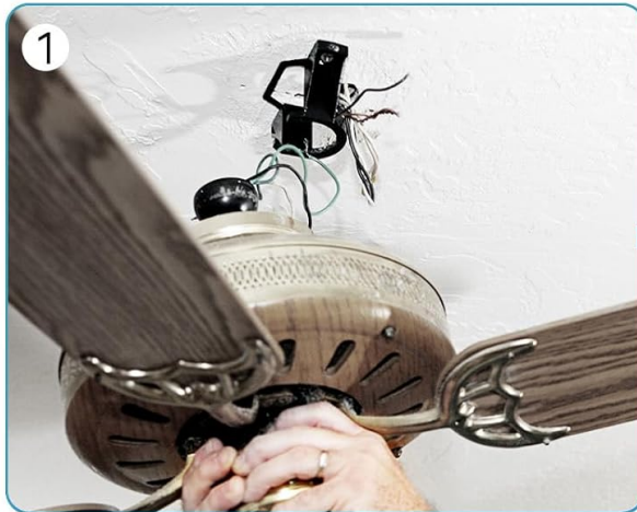
Disconnect the ceiling fan wiring
