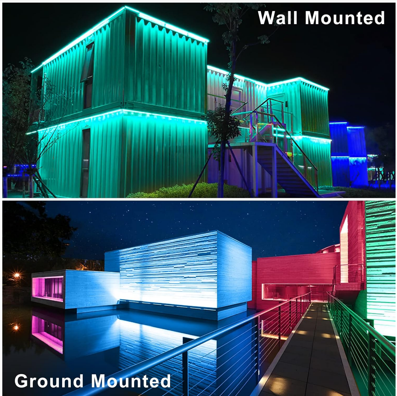
Image: Examples of wall-mounted and ground-mounted installations.
