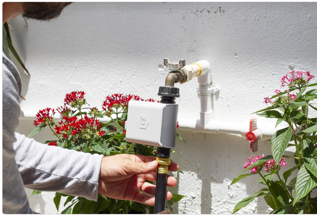
Image: Proper installation of the B-hyve timer on a hose faucet.
