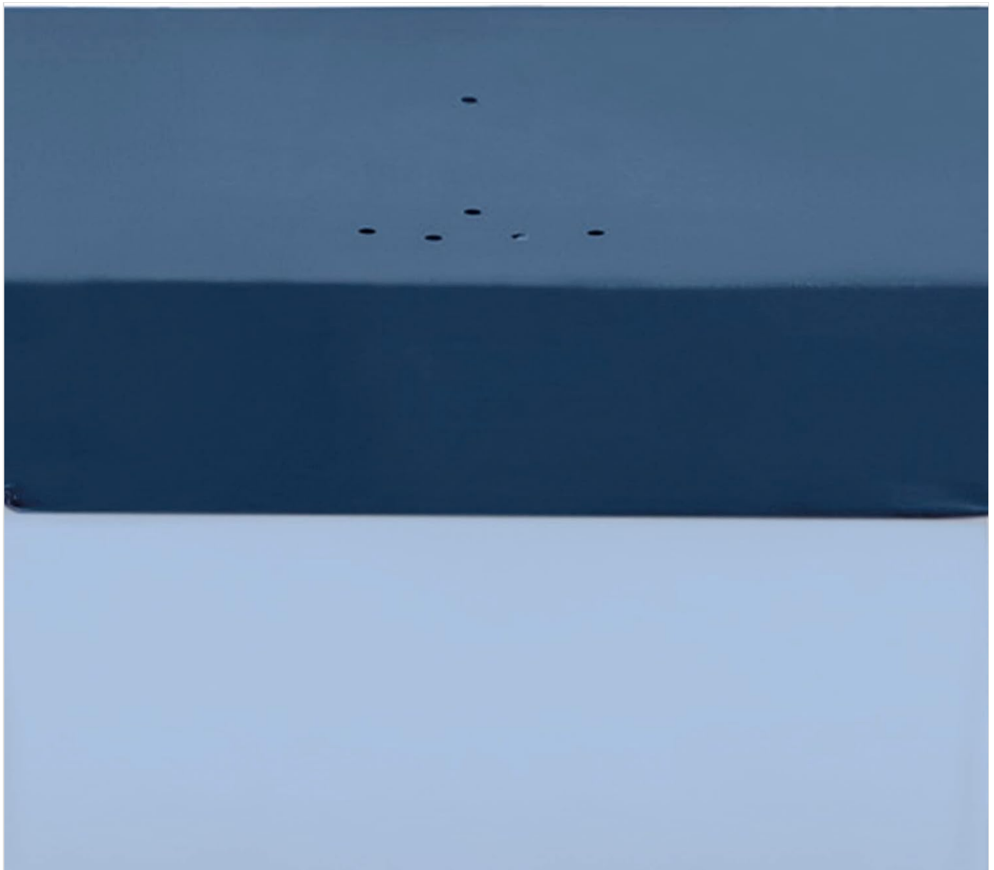
Image: Detail of the drainage holes on the pool cover, designed to prevent water accumulation.
