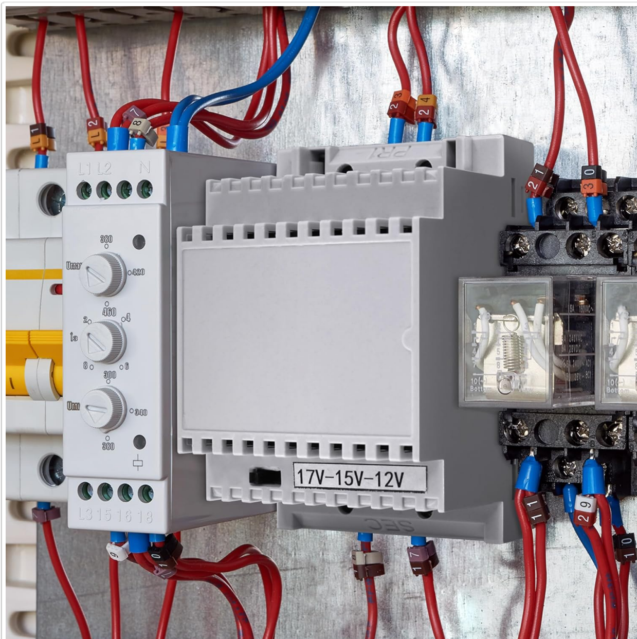
Figure 2: DIN Rail Transformer installation example.
