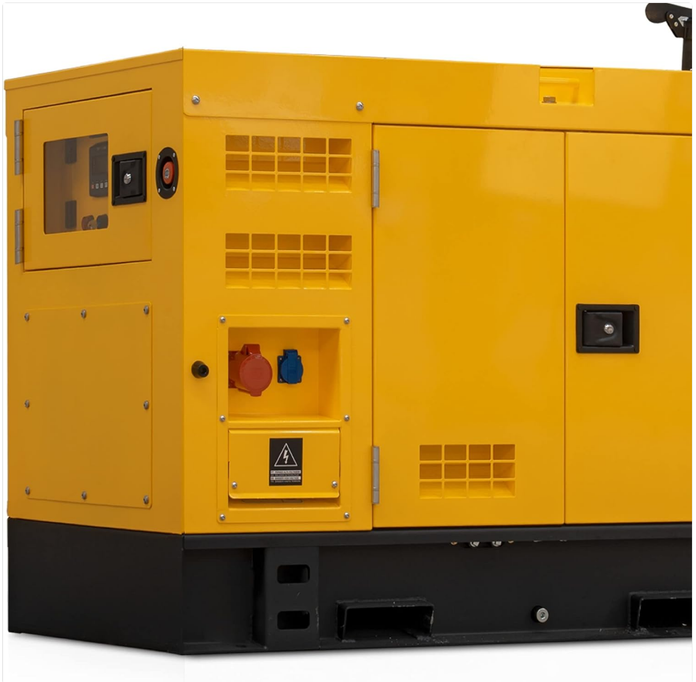
Figure 2: Close-up view of the generator's control panel and power outlets, including the single-phase (blue) and three-phase (red) receptacles, and the warning label.
