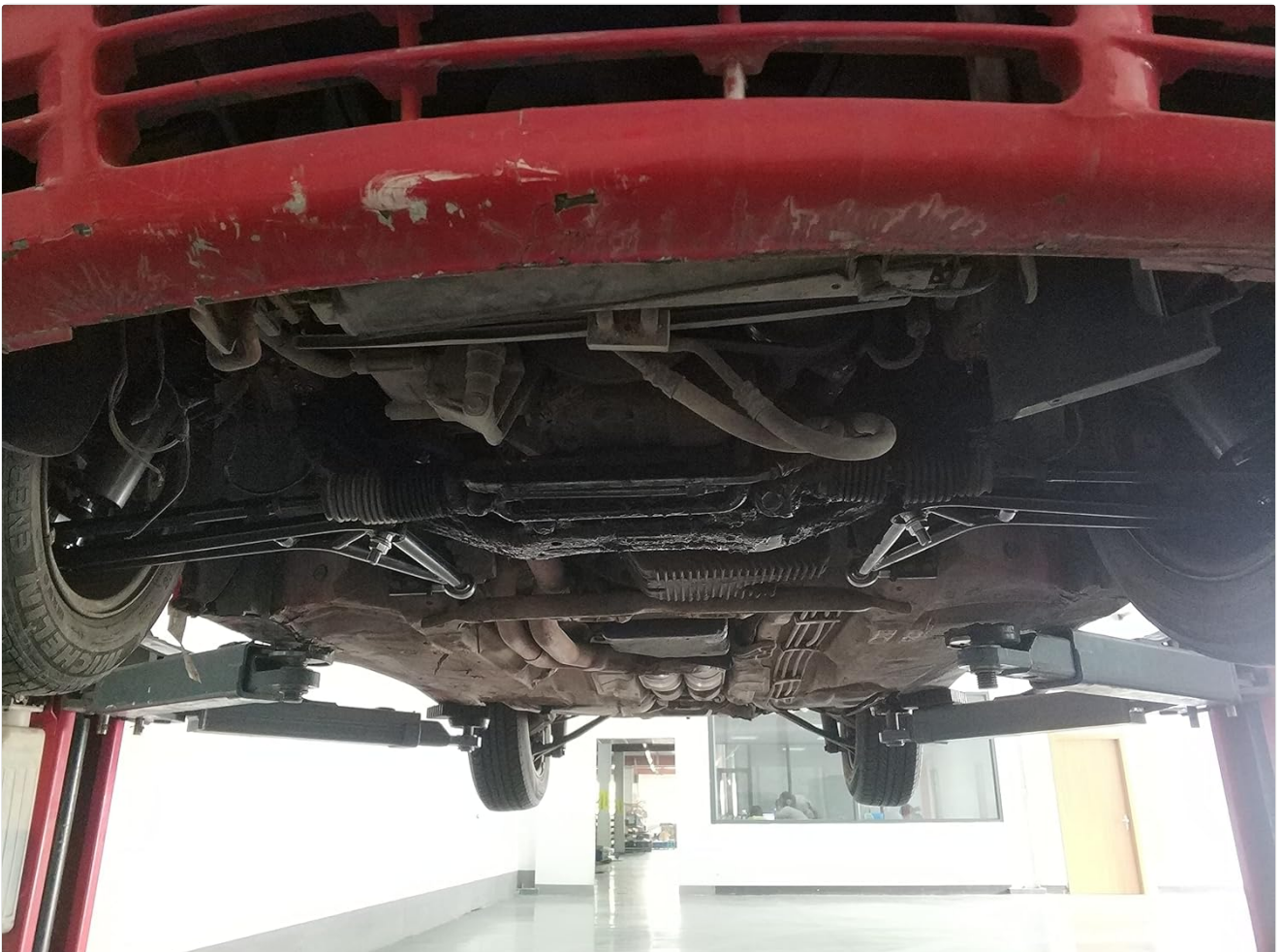
Image 4.1: A vehicle on a lift, illustrating the area where the control arms are installed.
