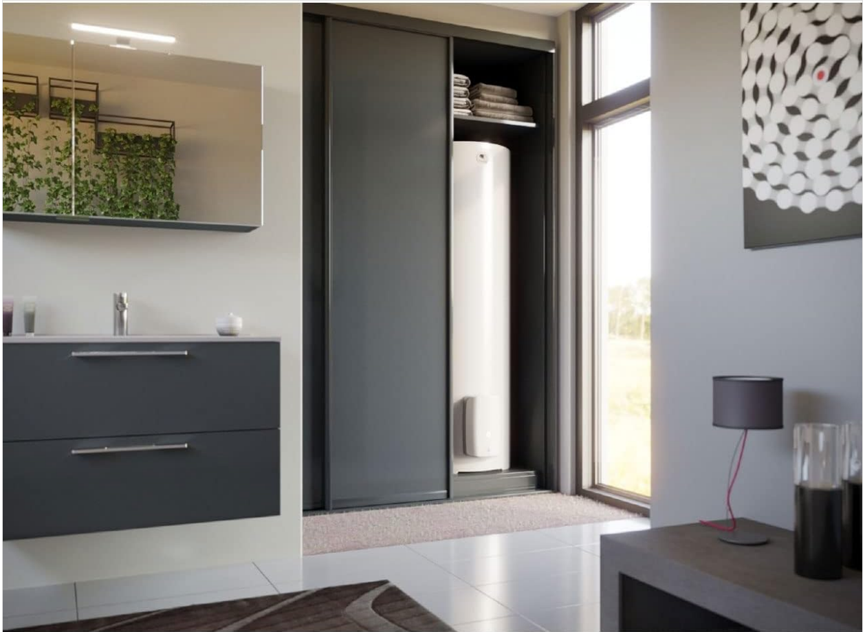
Figure 3.4: Installed Unit. An example of the water heater installed in a typical utility or storage space, demonstrating its vertical orientation and integration into a home environment.
