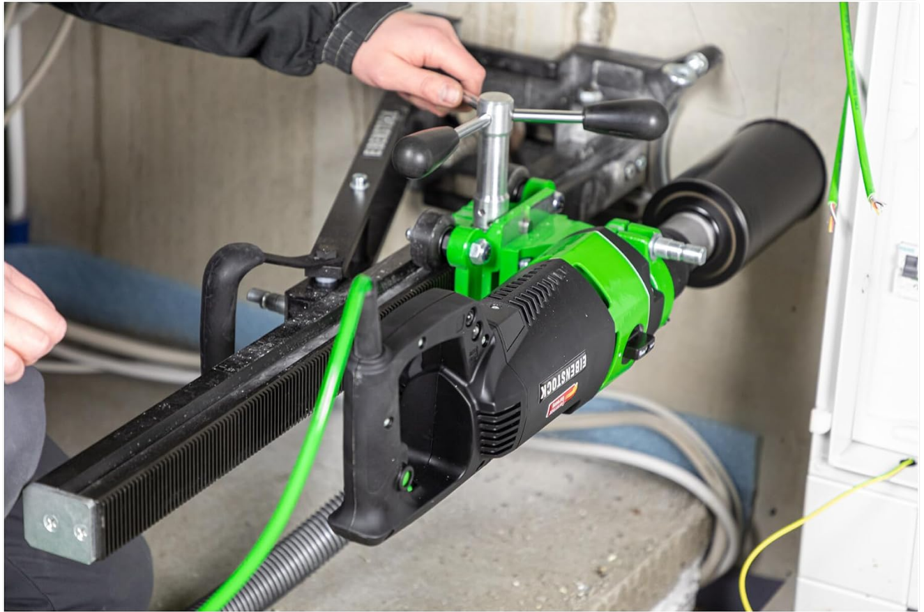
Figure 2: The ESD 162 drill securely mounted on a drill stand, ready for precise core drilling into a concrete wall. This setup enhances stability and accuracy.
