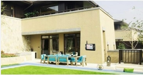
The launcher is mounted on the wall
