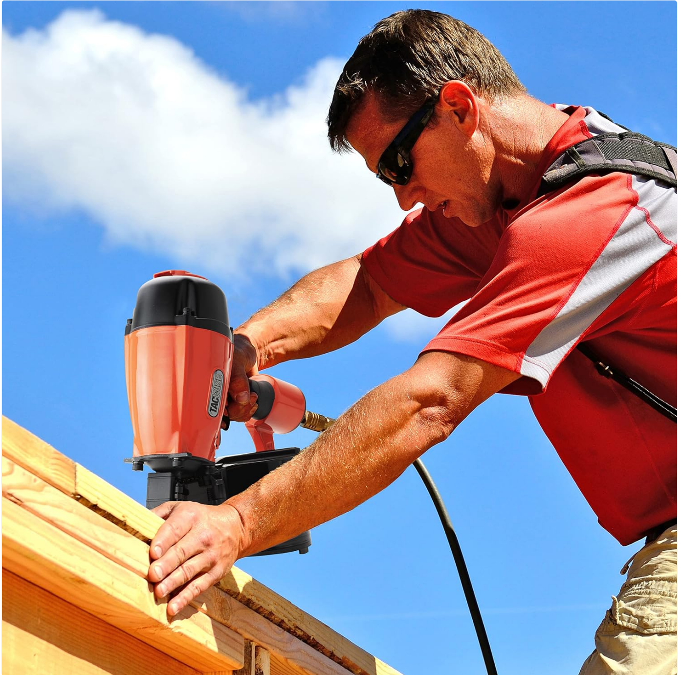
Figure 5.1: An operator demonstrating the use of the JCN90V nail gun in a construction setting, highlighting its application in timber framing or similar tasks.
