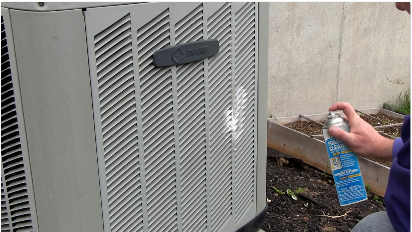
Image 4.1: Demonstrating the application of coil cleaner on an outdoor HVAC unit.
