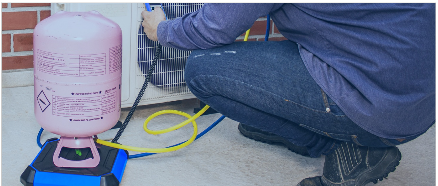
Image: The Xetron SRC-400 scale features a high-performance chip for excellent resolution and accuracy, with specifications listed as 0.011 lbs resolution, 220 lbs capacity, and \pm 0.05\% rdg + 0.022 lbs accuracy.
