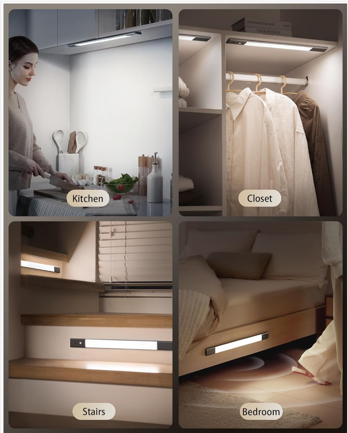
Image: Examples of EZVALO lights installed in different household areas, including under kitchen cabinets, inside a closet, on stair risers, and under a bed, demonstrating their versatility.
