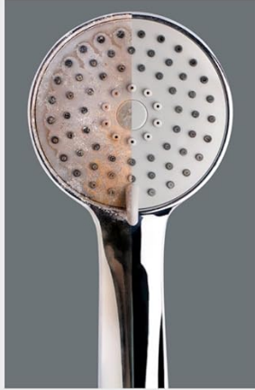
Scaling of Hot Water Appliances
