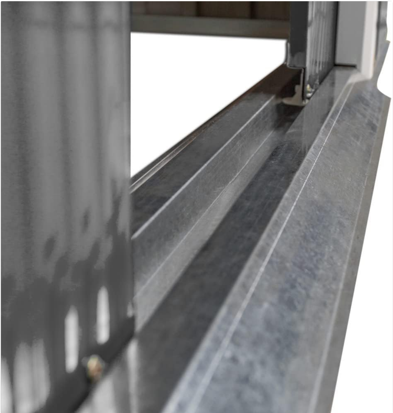
Figure 4: Detail of the lower sliding door track, showing the mechanism that allows the door to open and close smoothly.
