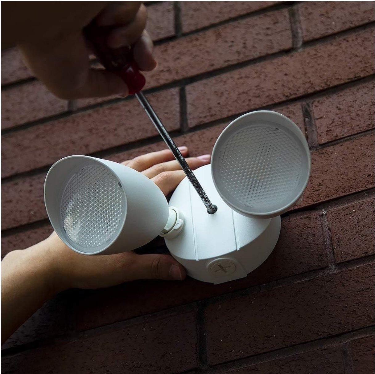
Image: A person using a screwdriver to secure the flood light base to a brick wall during installation.
