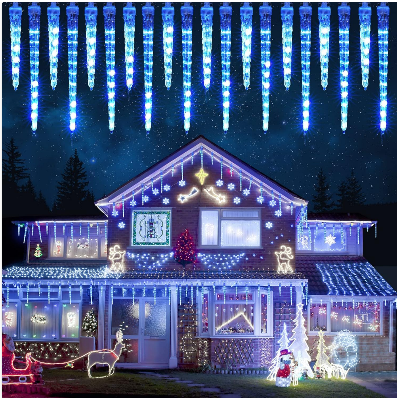
Image 1: Joomer Icicle Christmas Lights installed on a house.
