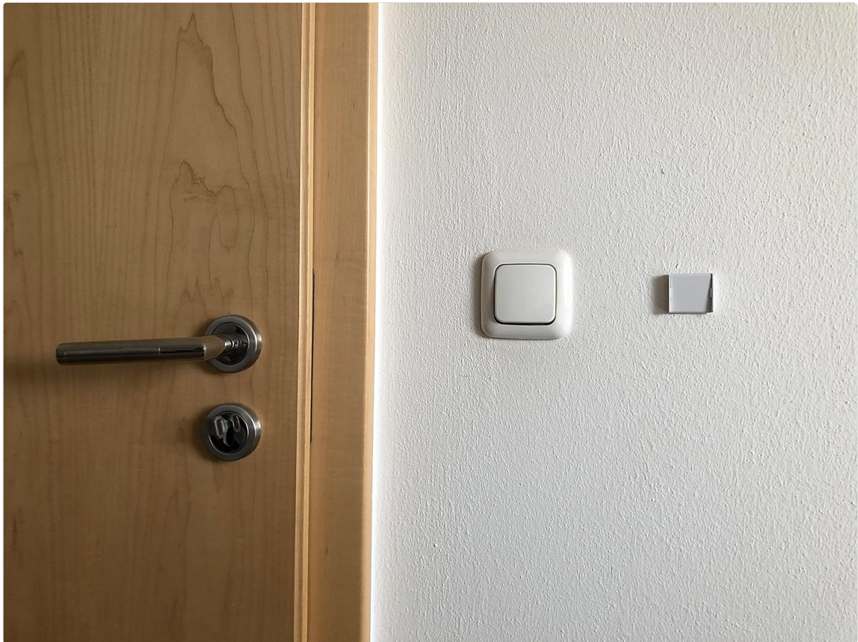
Image 4.1: This image shows a white wall next to a wooden door and a light switch. To the right of the light switch, the small, grey base of the remote control wall mount is temporarily placed against the wall, indicating where it will be installed. This step involves marking the precise drilling points for the screws.
