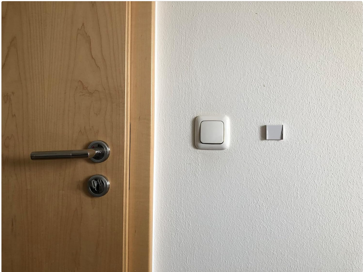
Image 4.2: The image displays the white wall mount base, now securely fastened to the wall using screws and anchors. It is positioned to the right of a standard light switch, demonstrating the completed attachment of the base component before the cover is applied.
