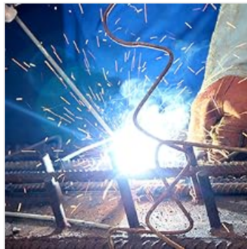
Figure 5.6: Example of MMA (stick) welding in progress.
