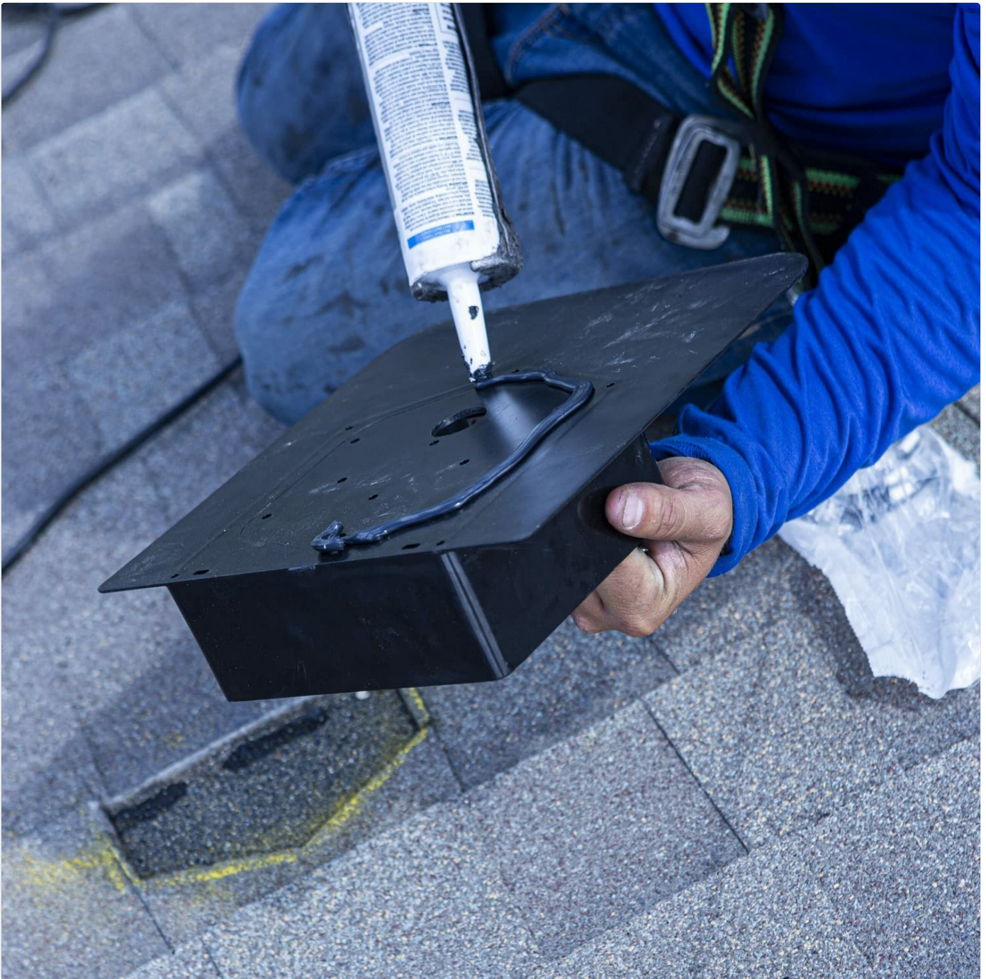
Figure 5.2: Applying sealant to the junction box base for a watertight seal.
