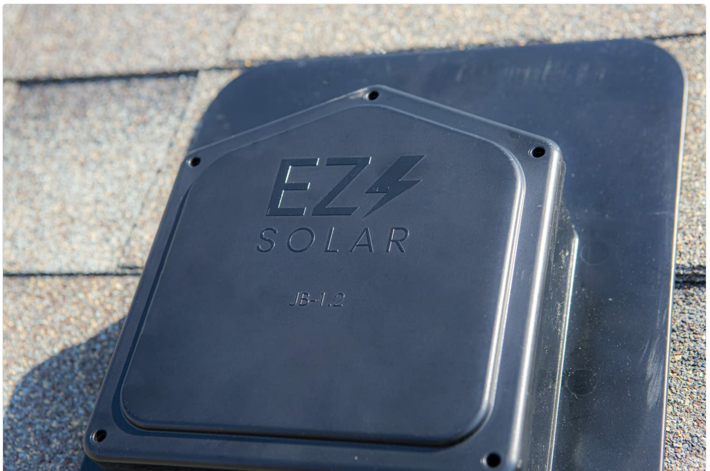
Figure 5.3: The JB-1.2 junction box securely mounted on a shingle roof.
