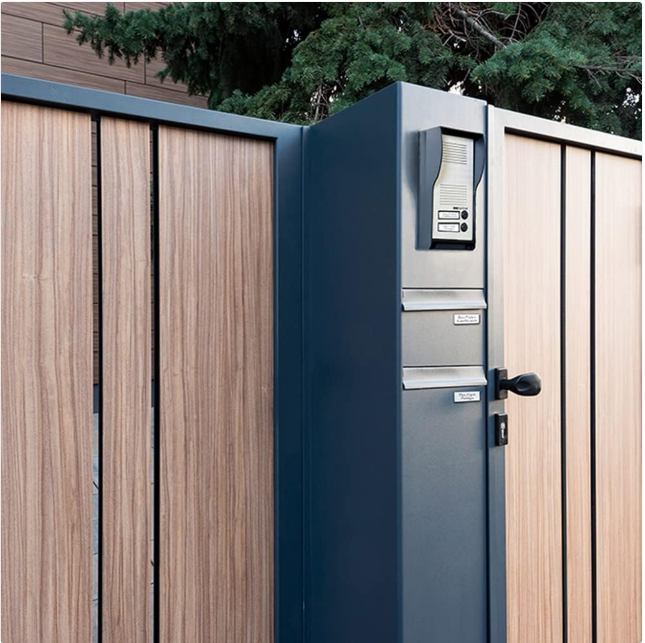
Figure 3: Example of Outdoor Street Plate Installation on a Gate.
