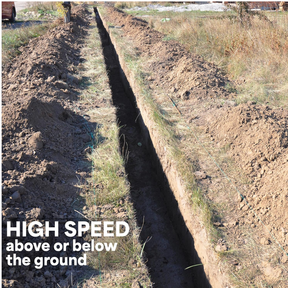
Image: A prepared trench in an outdoor setting, illustrating the method for direct cable burial.
