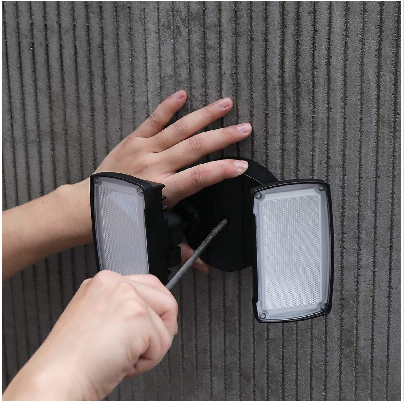
Figure 2: Installation of the floodlight on a wall.
