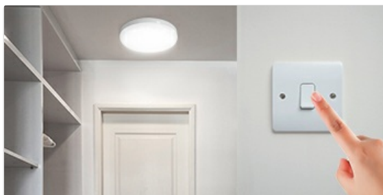
Image: The ceiling light is operated via a standard wall switch.
