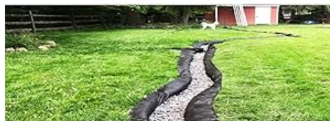
Image 4.2: Illustration of ground stabilization using geotextile fabric as a separation layer.
