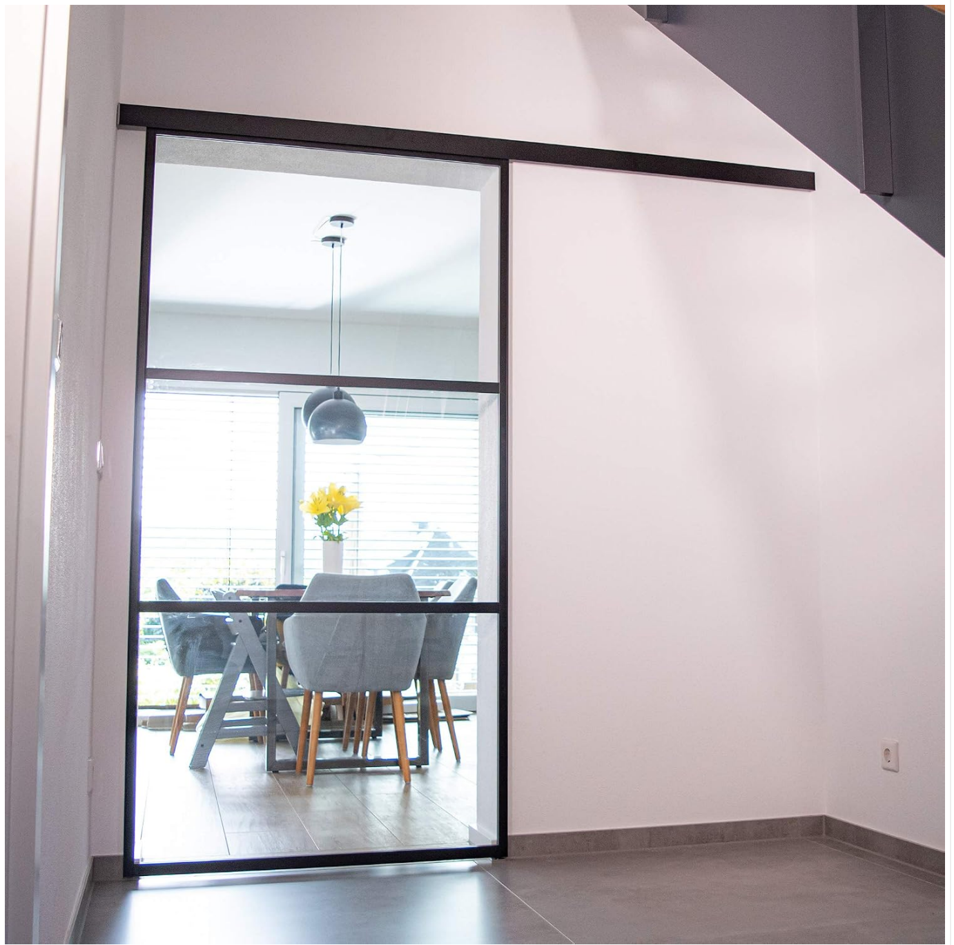
Figure 4.2: Example of a fully installed sliding door.
