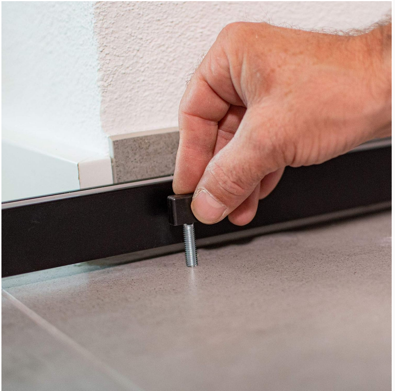
Figure 4.4: Installing the floor guide pin.
