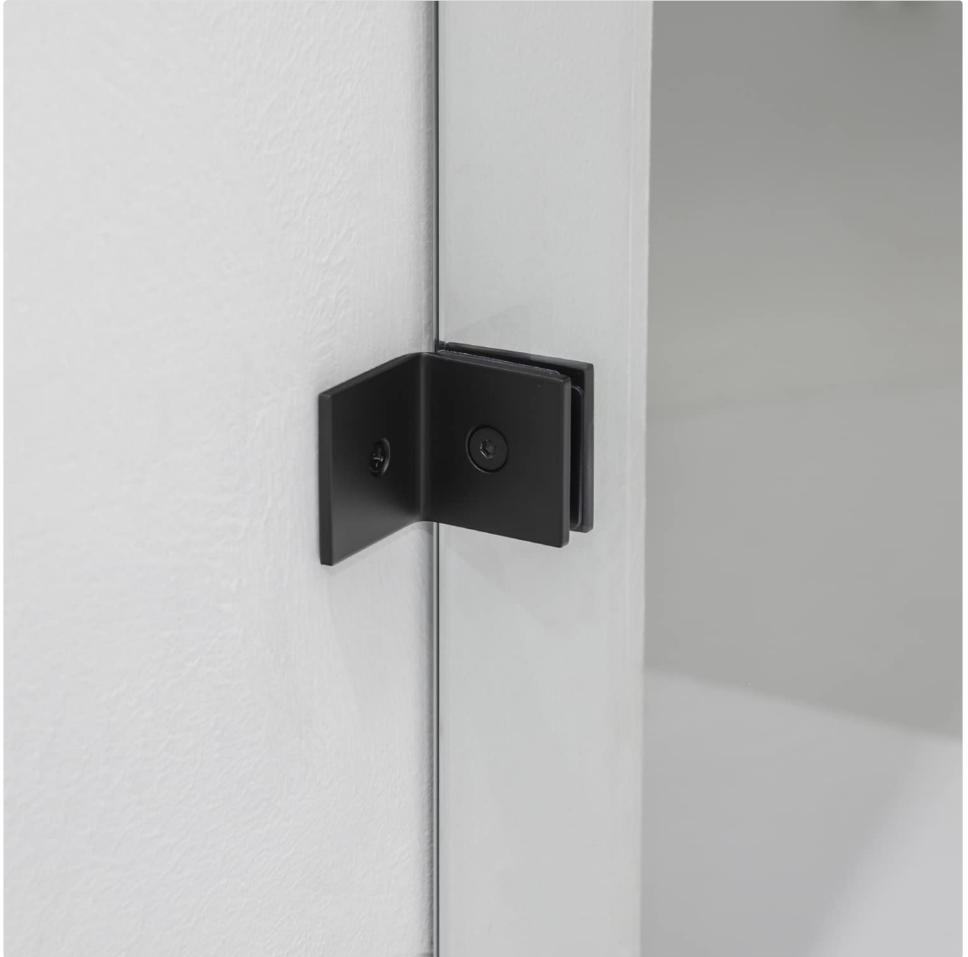
Figure 4.1: Secure the stainless steel wall brackets firmly to the wall. These brackets reinforce the side panel, ensuring stability.
