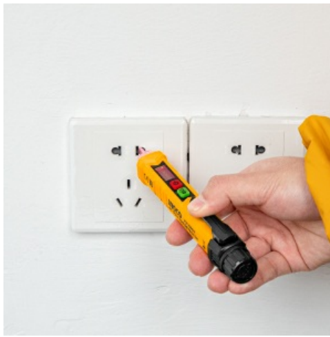
Image 5.1: Non-contact voltage detection at an electrical outlet.
