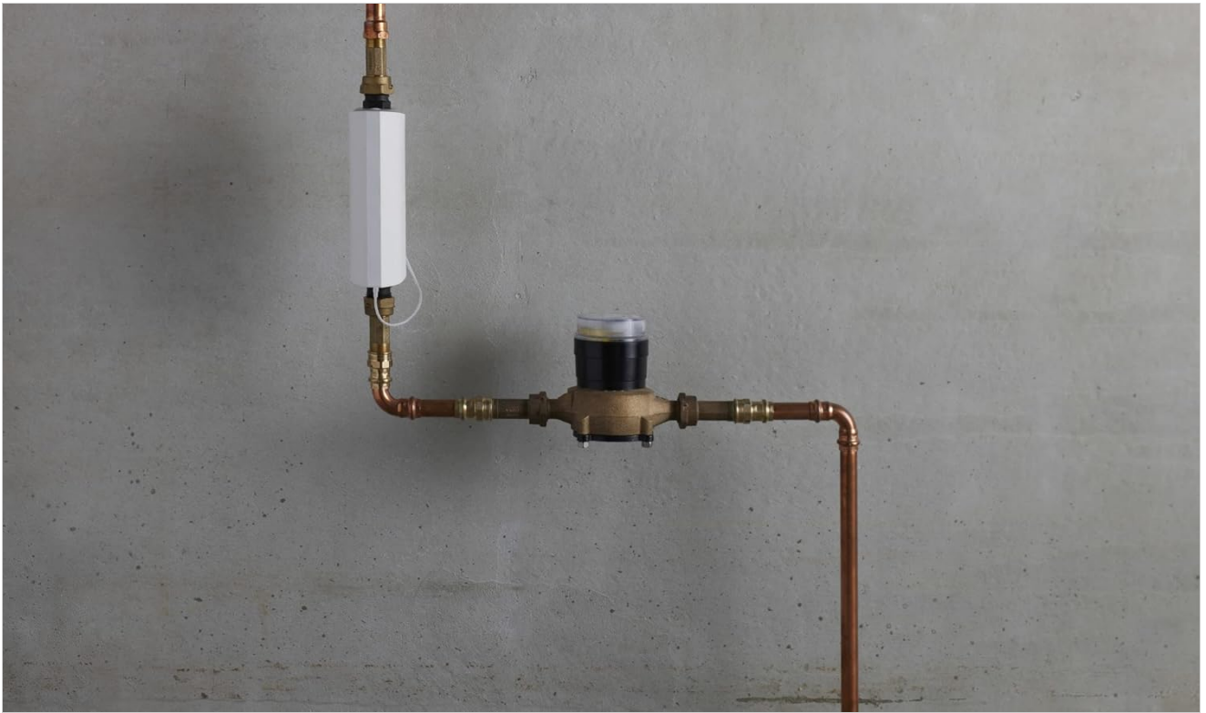
Figure 5.3: The H2Wise+ unit installed on a main water pipe, demonstrating a typical setup.
