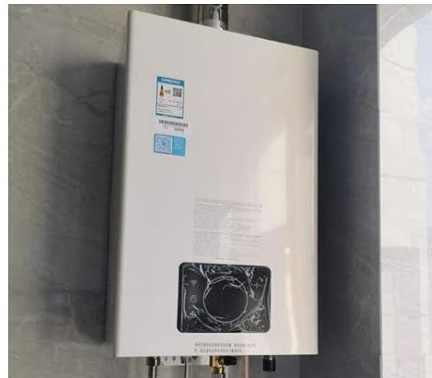
GAS WATER HEATER
