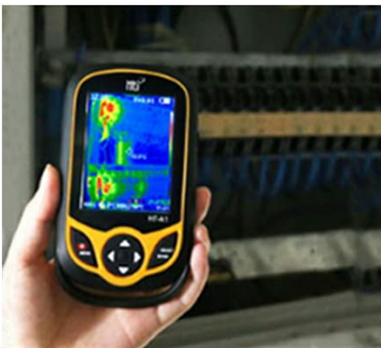
Electric box check
