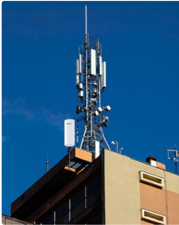
Figure 6: Example of pole mounting for the CPE451.
