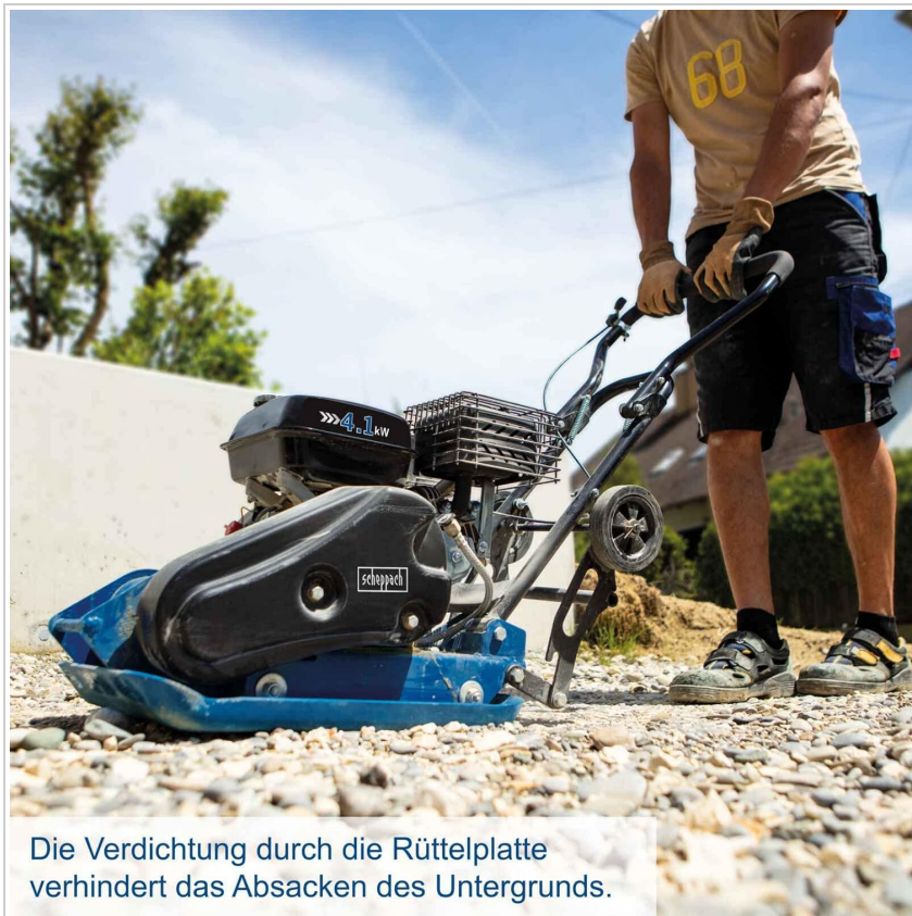
Image 2: The vibratory plate compacts the subsoil to prevent subsidence.
