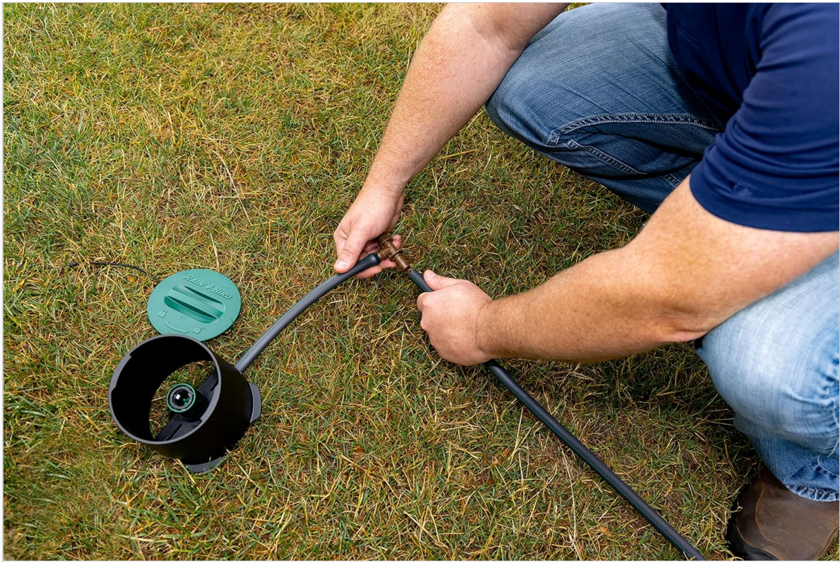
Image: Connecting the distribution tubing to the Click-N-Go housing.
