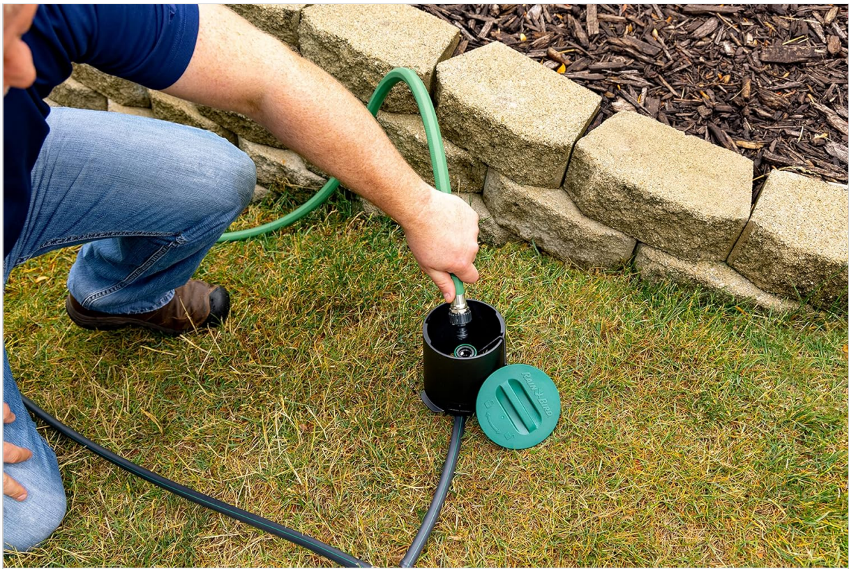
Image: A person connecting a sprinkler head to the distribution tubing.
