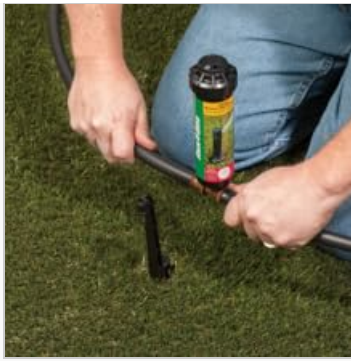
Image: A person burying the distribution tubing in a shallow trench.
