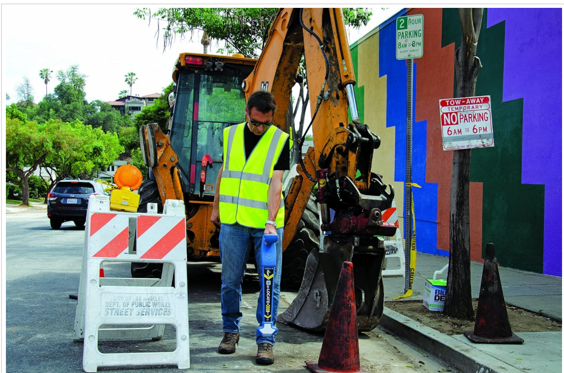
Image: An operator using the u-LOCATE Receiver in an urban environment near an excavation, highlighting its use in complex settings.
