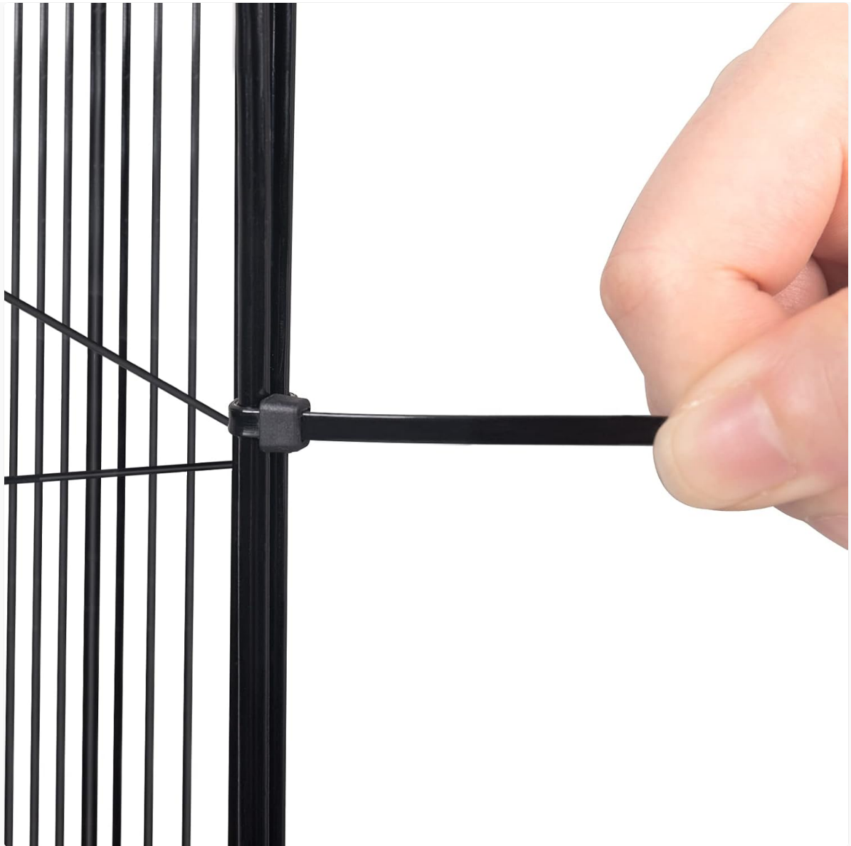
Image: Reinforcing connections with cable ties.
