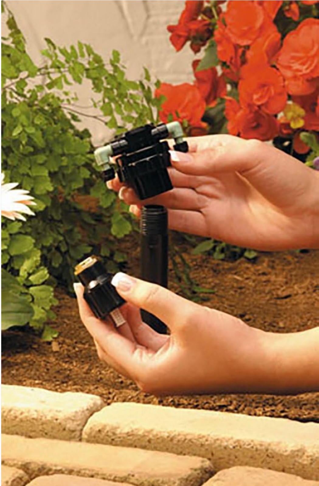
Figure 3: Adjusting the flow control on the manifold.
