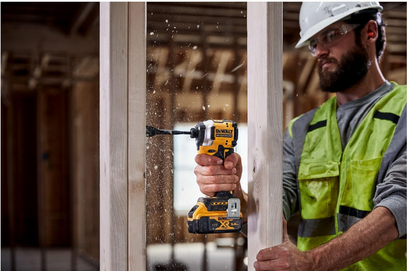
Figure 6: The impact driver driving fasteners into wood framing.
