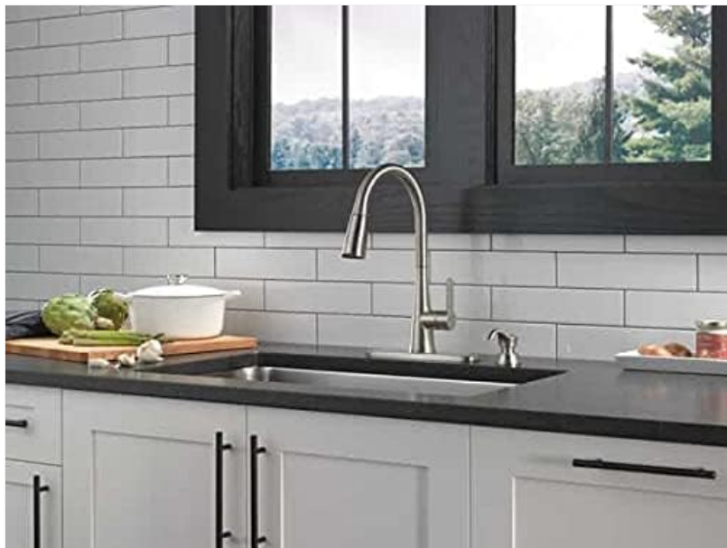
Image: The Delta Greydon Faucet installed in a kitchen, showcasing its design and finish.
