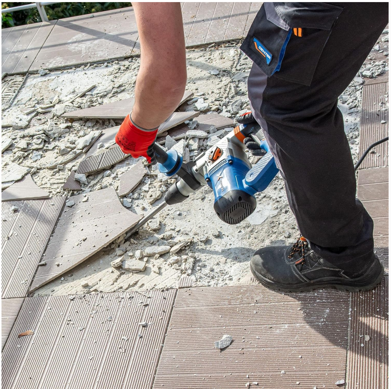
Figure 8: An operator using the hammer drill to efficiently remove floor tiles, utilizing the chiseling function.
