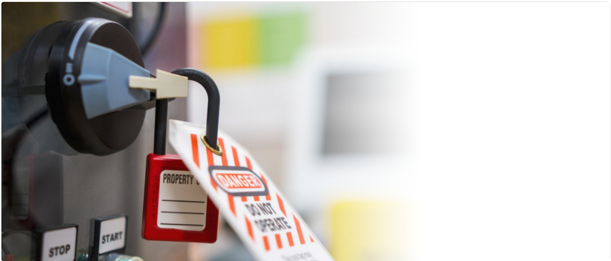
Image: An industrial setting with a safety padlock on equipment, emphasizing the importance of safety procedures like lockout/tagout before working with electrical components.
