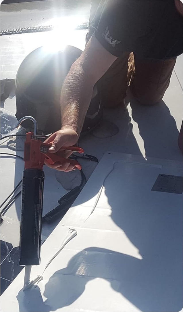
Image 3.1: Examples of flexible solar panel installation, showing adhesive mounting on a roof and hanging on a vehicle side.
