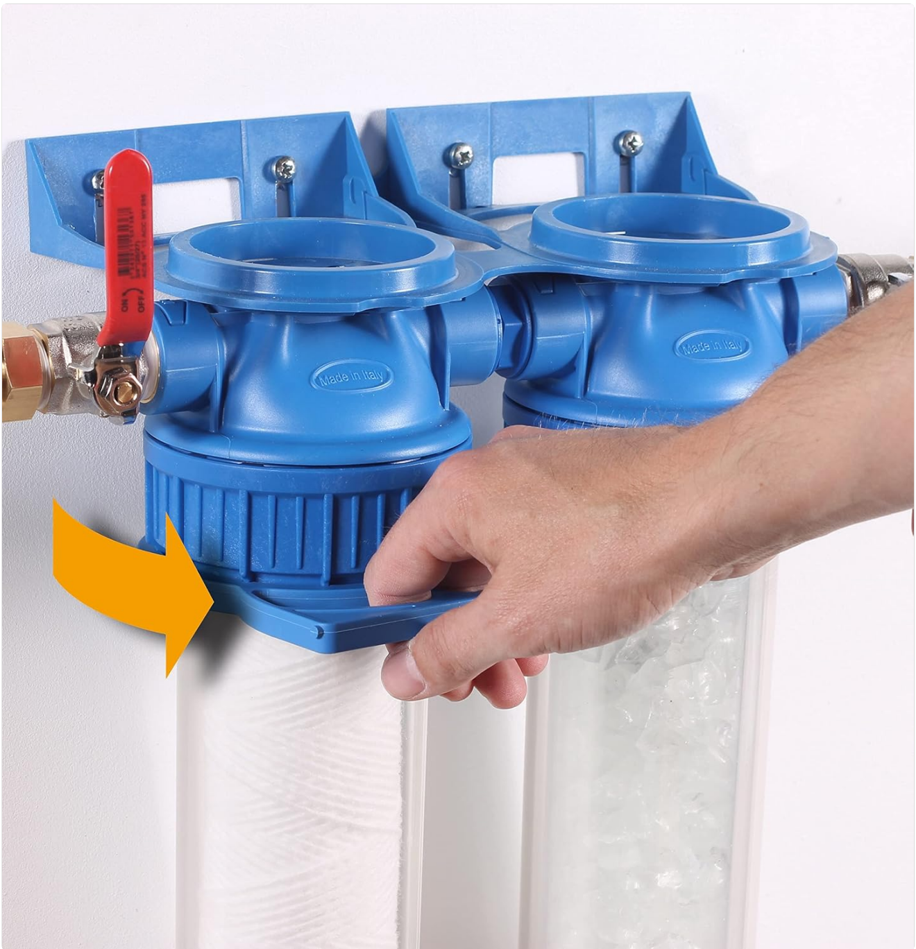
Image 6.3: Tightening the filter housing after cartridge replacement.
