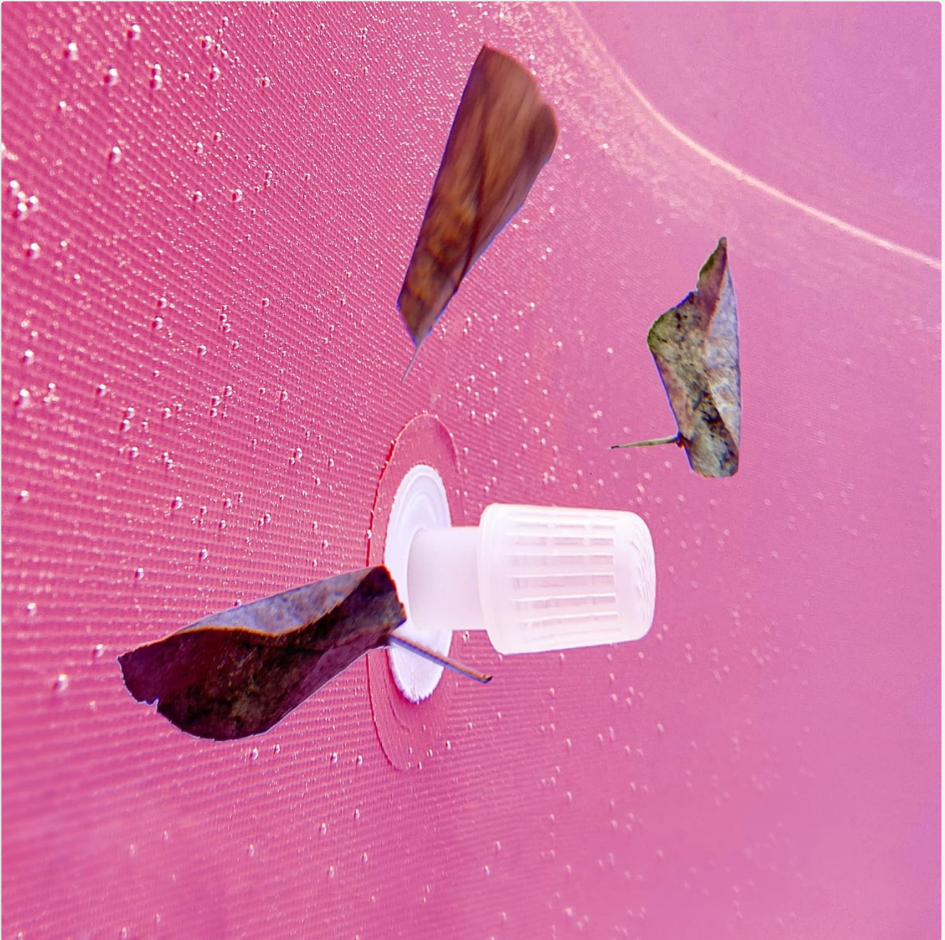
Image 5.1: Close-up view of the pool's drain/inlet port, illustrating where debris might accumulate and the connection point for drainage.
