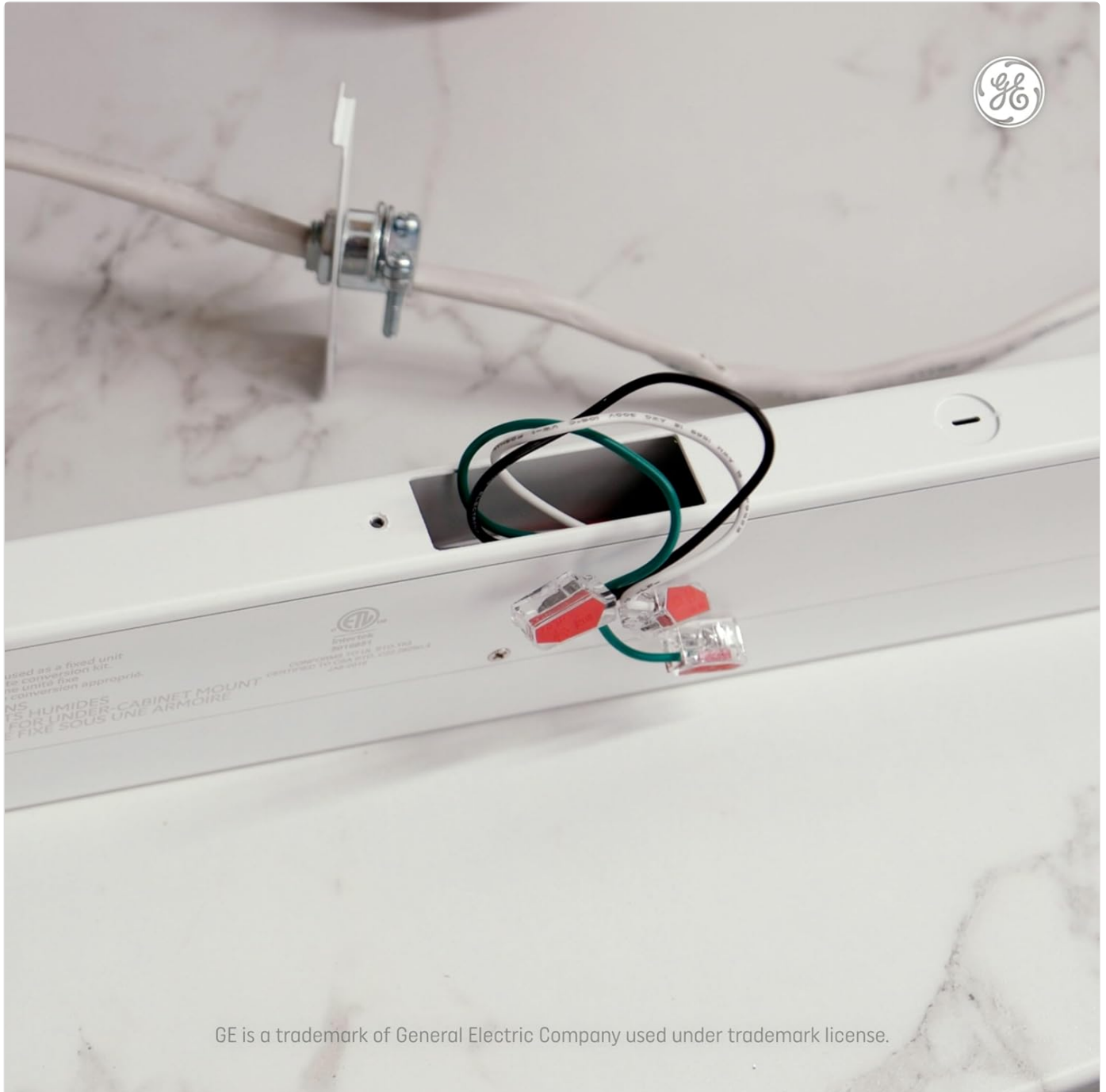
Image: A close-up showing electrical wires being connected with wire nuts, illustrating the direct wire installation method for the undercabinet light fixture.
